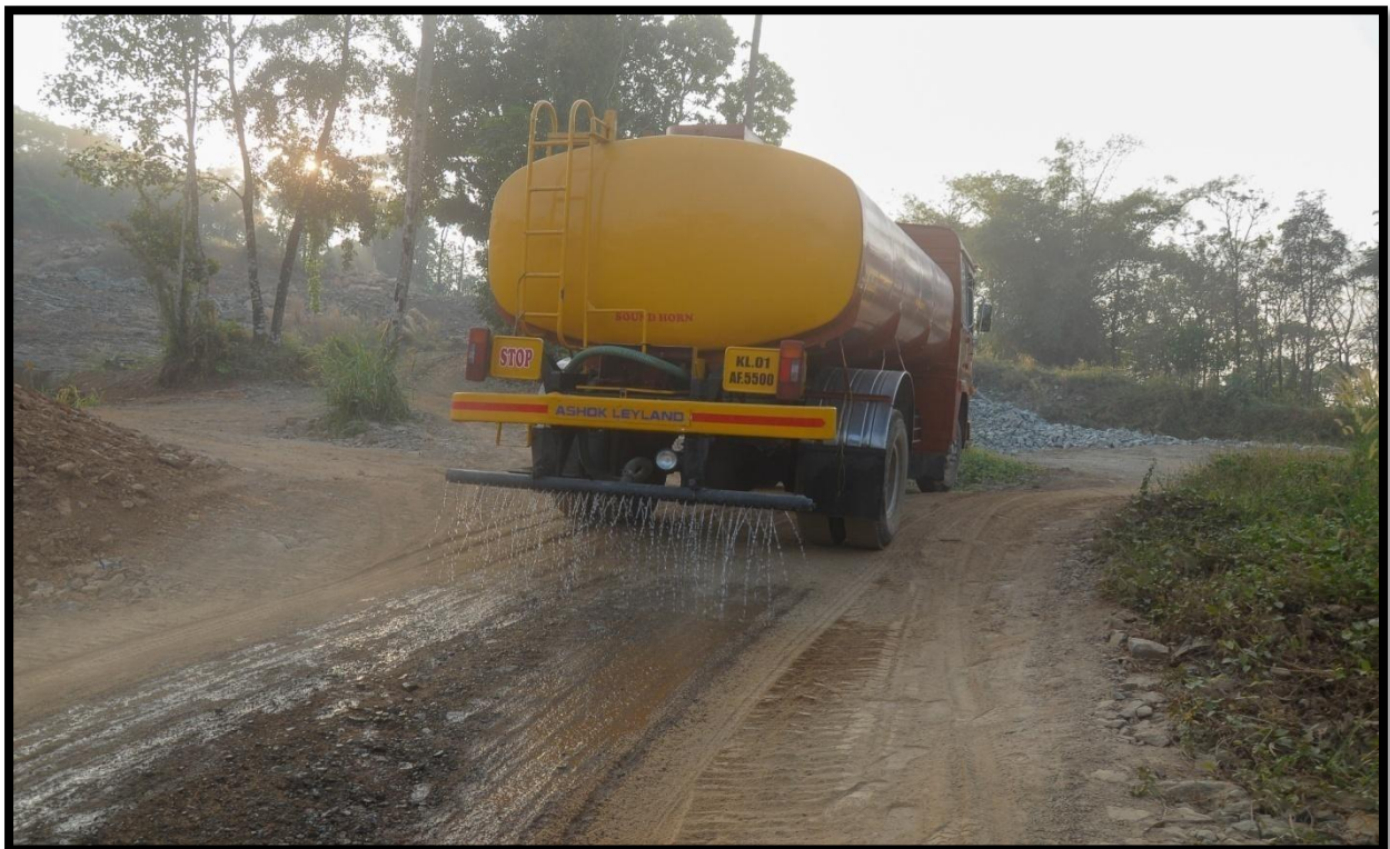
Water spraying using tanker vehicle
